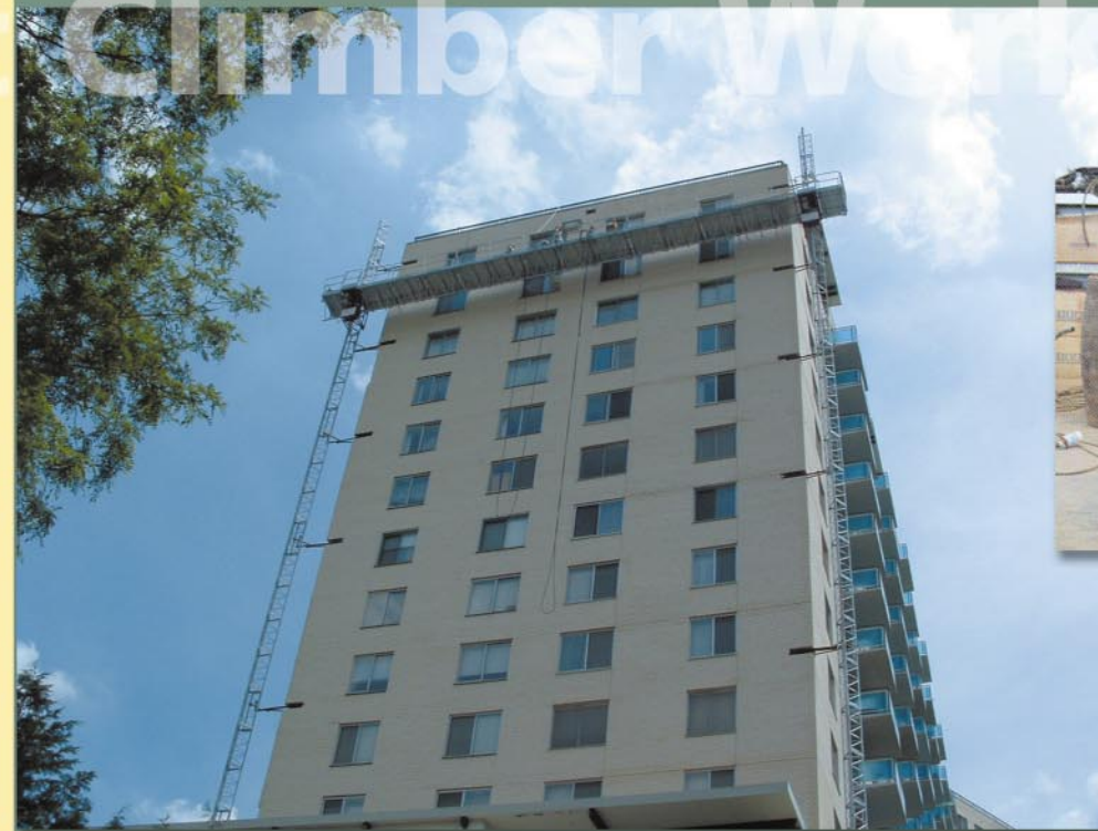
All structural parts are hot dip galvanized.
