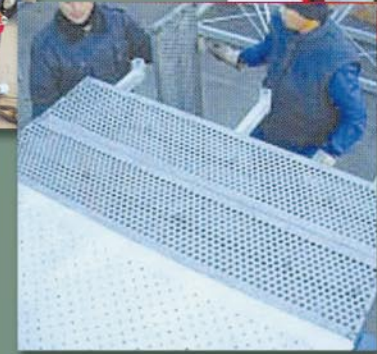
All structural parts are hot dip galvanized.
